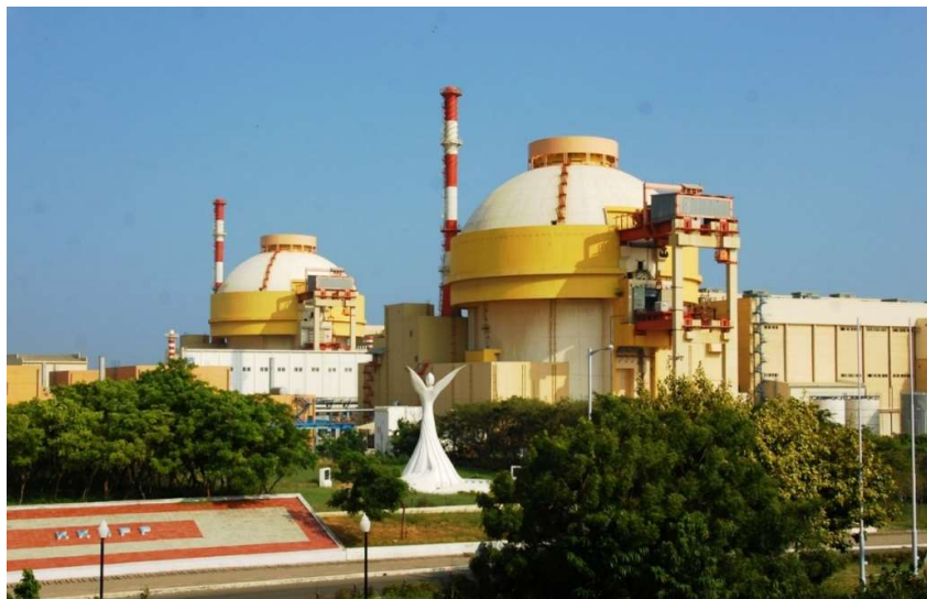
Figure 9-4: Kudankulam Nuclear Power Plant (Ref. 21)
