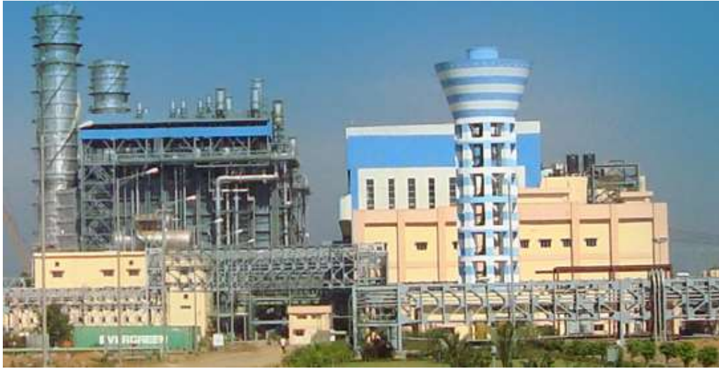
Figure 3-5: Tripura Combined Cycle Gas Power Plant (ref 19)
