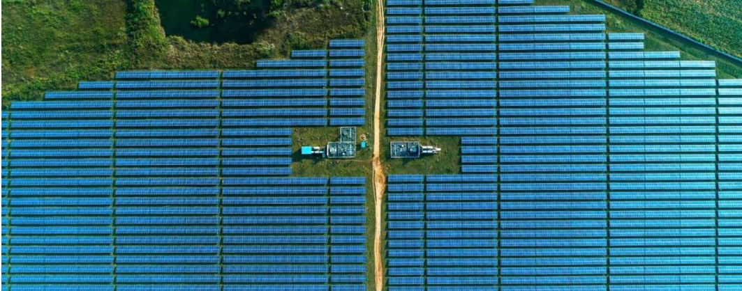
Figure 7-1: Utility scale PV plant
