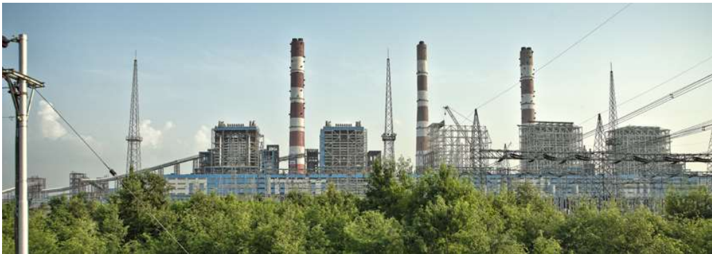
Figure 2-5: NTPC Barh Super Thermal Power Station (Ref. 17)
