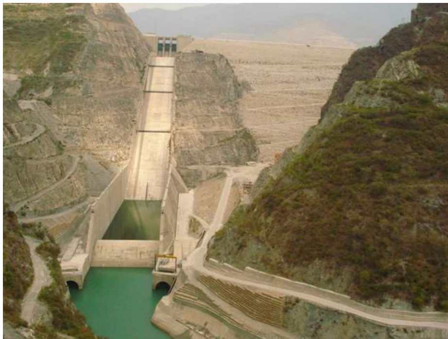
Figure 8-9 Tehri Dam, Uttarakhand (Ref. 17)
