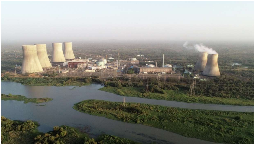
Figure 9-5: Kakrapar Atomic Power Station (Ref. 22)
