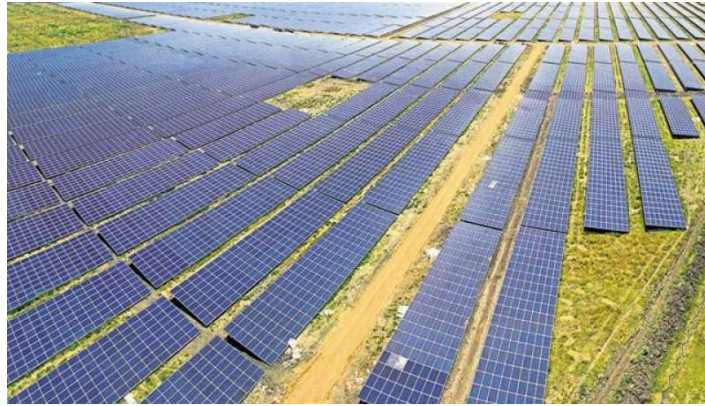
Figure 7-7: Rewa Solar Power Plant (Ref. 10)
