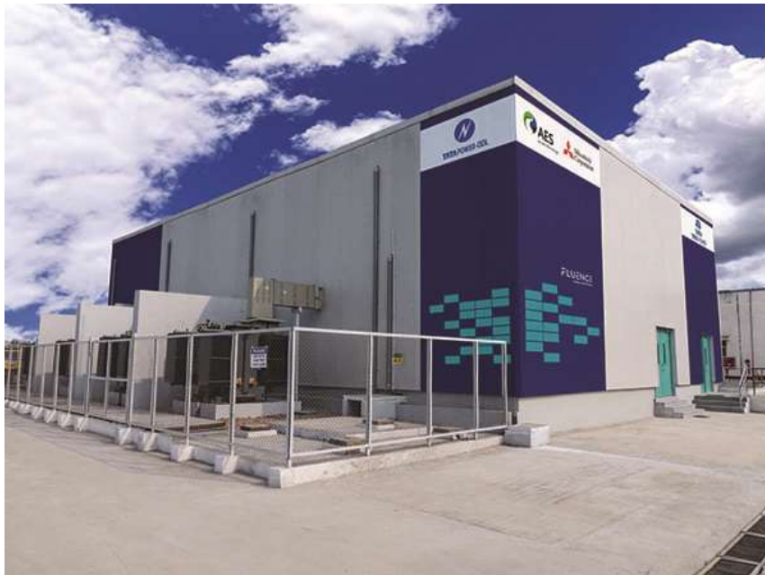
Figure 10-8: Rohini BESS, New Delhi (Ref. 46)
