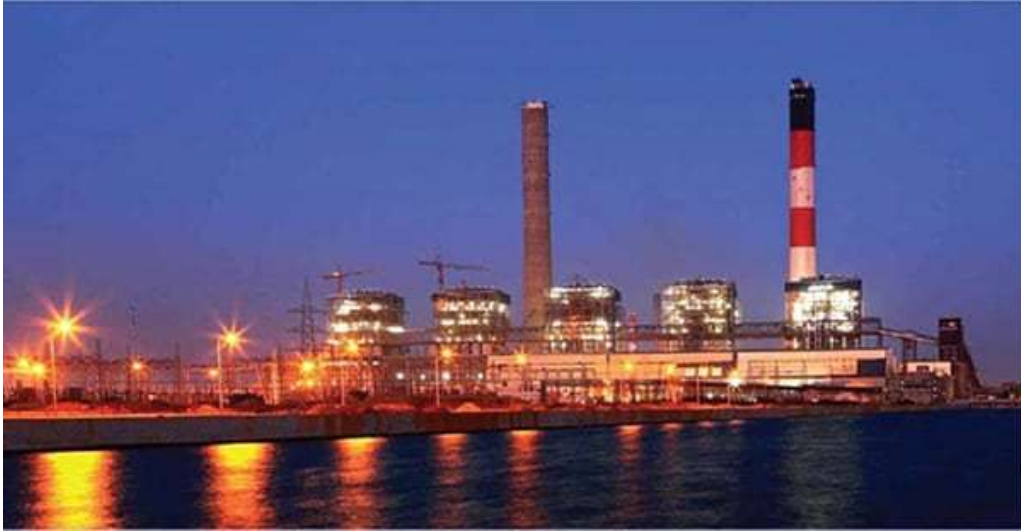
Figure 2-6 : Mundra Ultra Mega Thermal Power Station Gujarat (Ref. 18)
