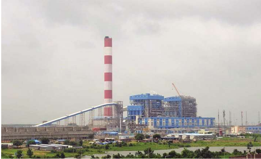
Figure 2-7: Khargone Power Plant (Ref. 19)
