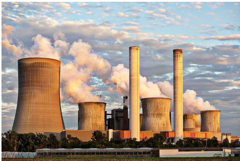
Figure 2-4: Vindhanchal Thermal Power Station, Madhya Pradesh (Ref. 16)
