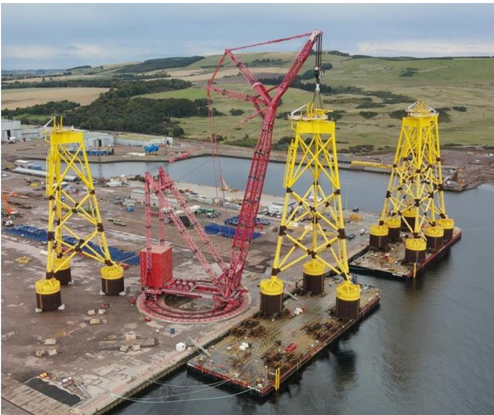
Figure 87: Loadout of jacket foundations by ring crane. Mammoet.
