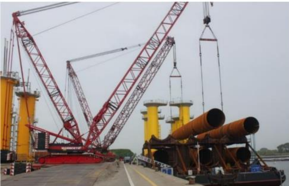
Figure 77: Loading of Monopile foundations and transition pieces
