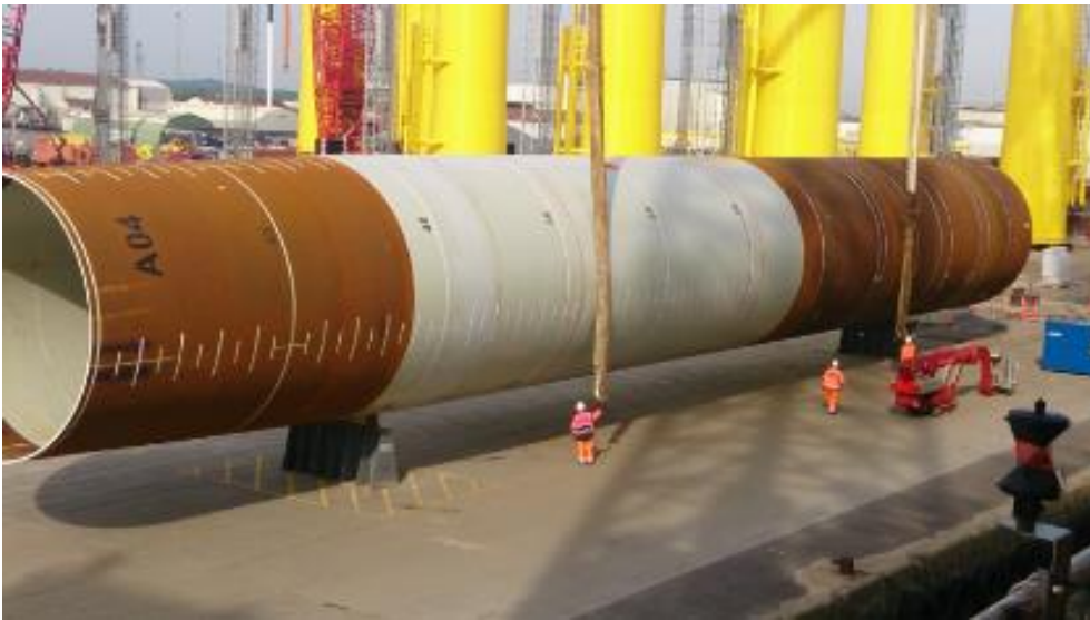
Figure 82: Monopile foundation on steel cradles prepared for loadout
