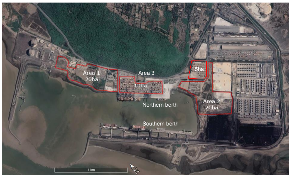
Figure 41: Hazira Port – Current port yards
