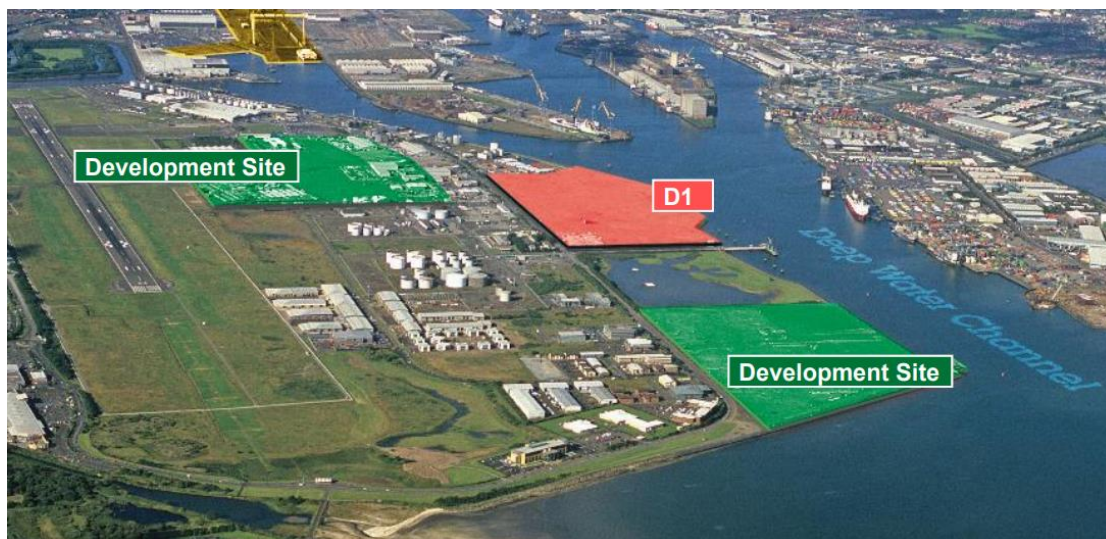
Figure 74: Case Study 3 – Offshore wind facilities at Port of Belfast
