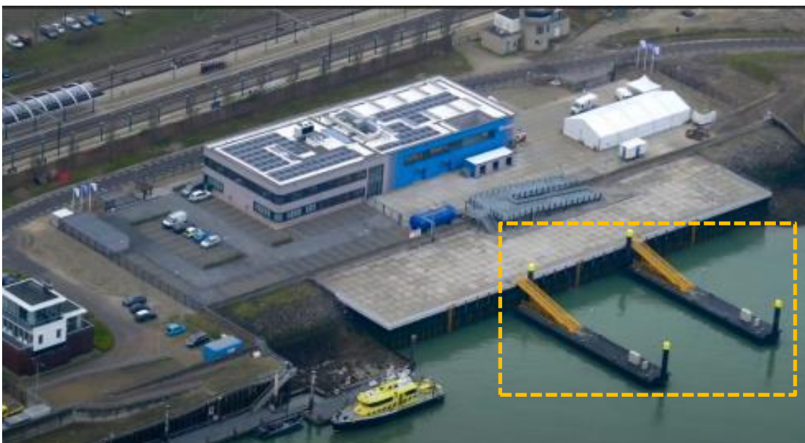
Pontoons highlighted within orange dashed area. Figure 14: Ørsted's O&M base at Vlissingen.
