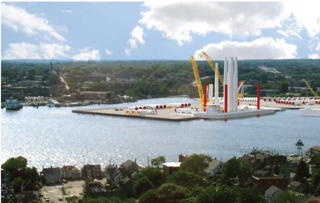
Figure 71: Case Study 1 – New London State Pier Infrastructure Improvement projects
