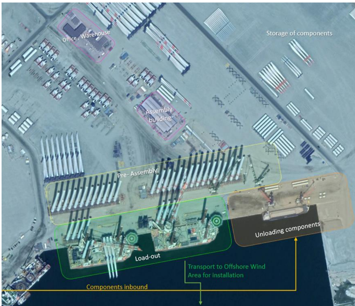
Figure 7: Typical layout for an installation port. (Esbjerg Port)
