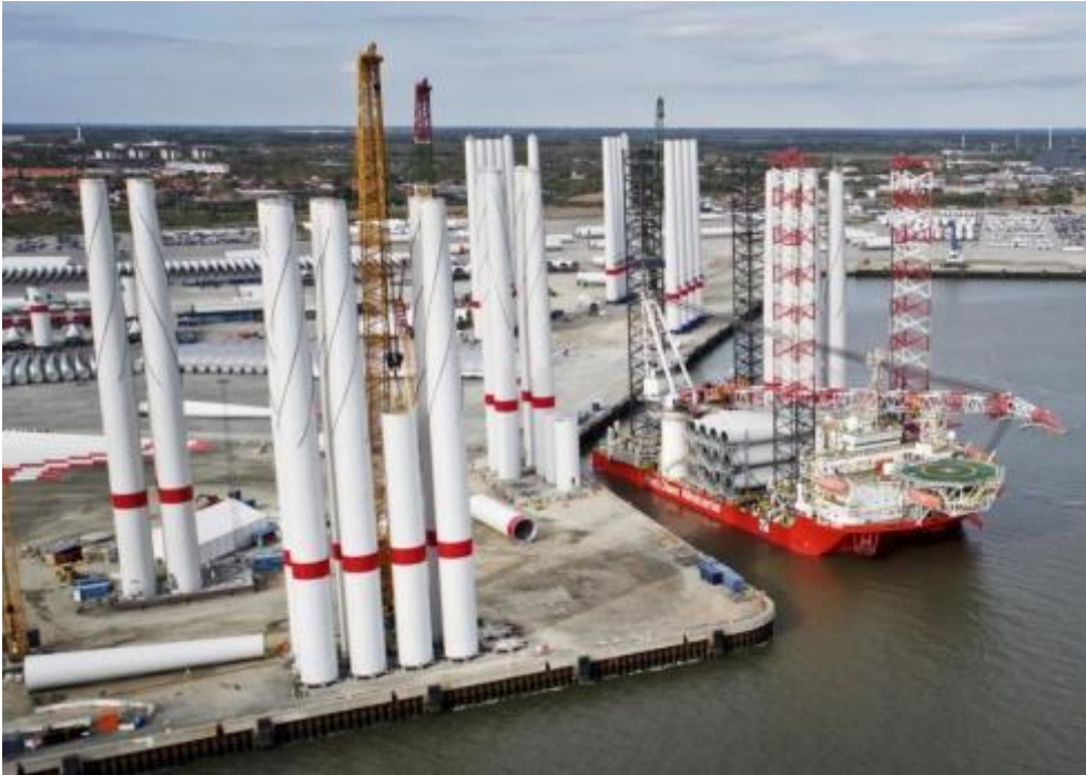
Figure 80: Tower assembly and loadout (source: Port of Esbjerg)
