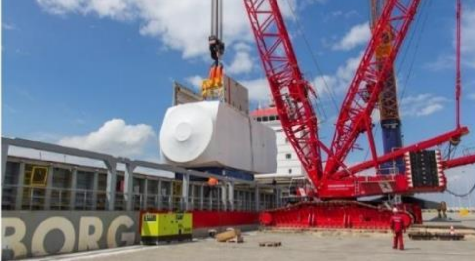
Figure 76: Figure Crawler cranes used in loadout of many major OWF components.
