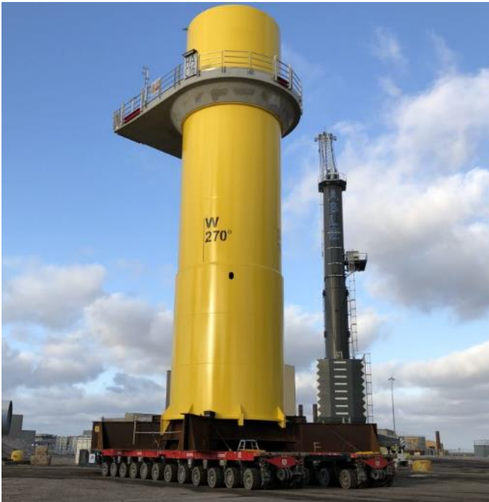
Figure 85: Transport of transition piece. Ableuk
