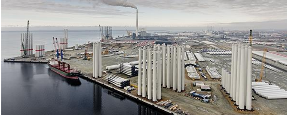
Figure 5-1 | Port of Esbjerg in Denmark load out facilities (Esberg)
